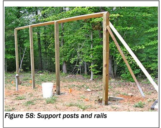
Figure 58: Support posts and rails
