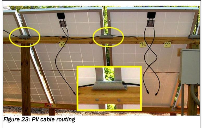
Figure 23: PV cable routing
