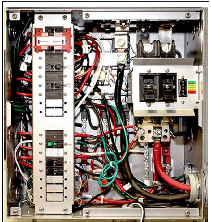
Figure 61: Load center for Radian inverter
