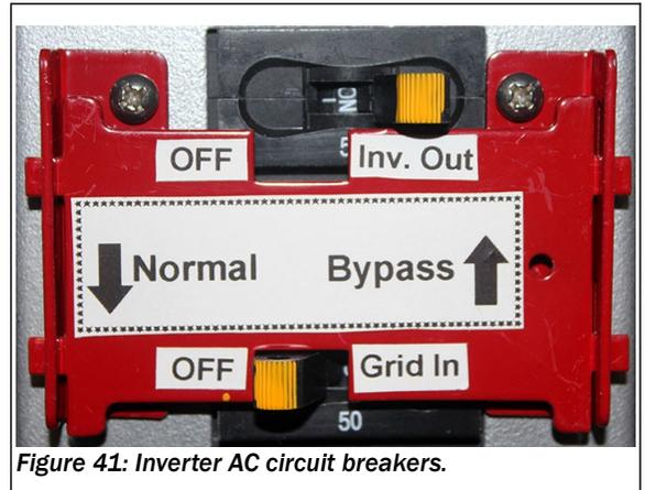
Figure 41: Inverter AC circuit breakers.
