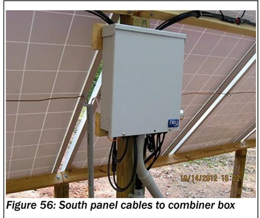
Figure 56: South panel cables to combiner box
