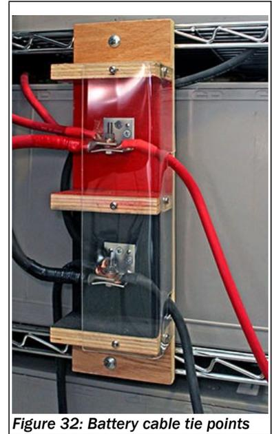
Figure 32: Battery cable tie points
