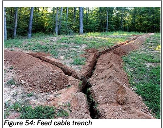
Figure 54: Feed cable trench
