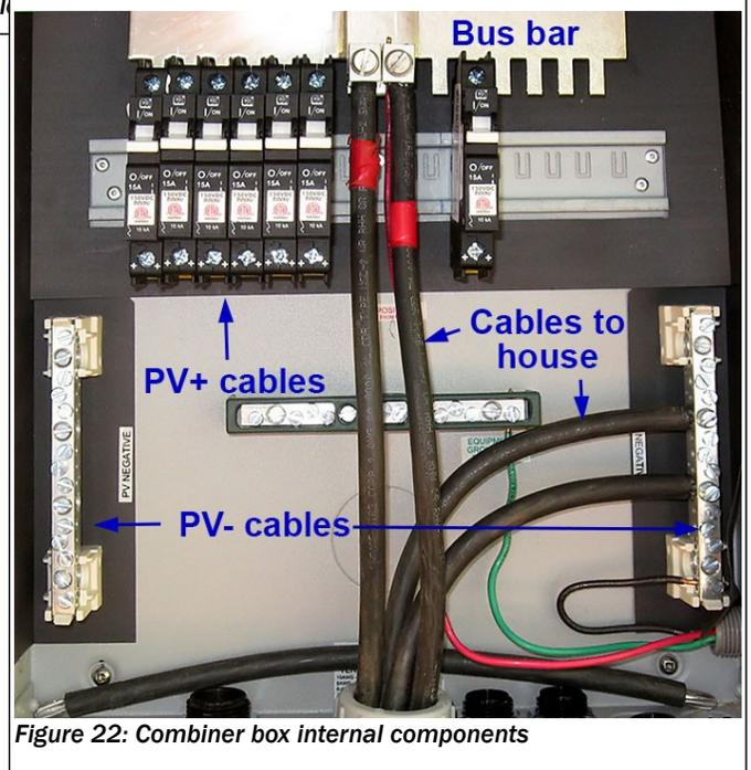
Figure 22: Combiner box internal components
