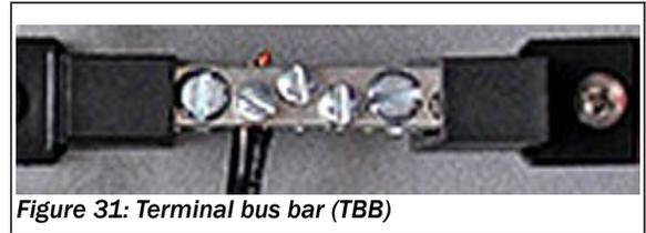
Figure 31: Terminal bus bar (TBB)
