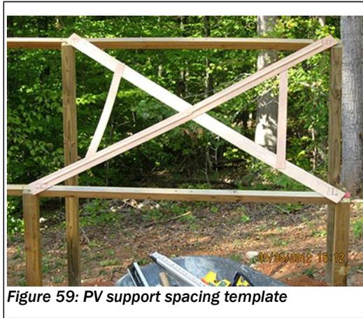
Figure 59: PV support spacing template
