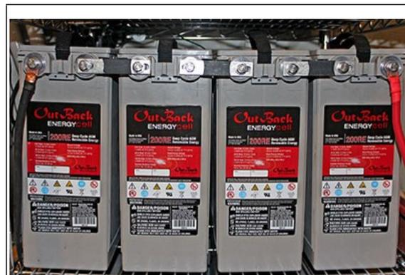
**Figure 6: String of four AGM batteries**
