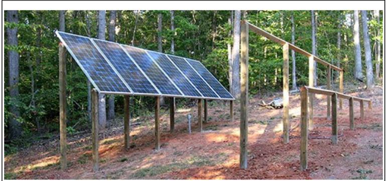
Figure 19: Wooden PV panel supports
