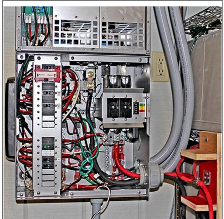
Figure 37: Load center installed beneath inverter
