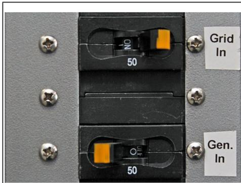
Figure 40: AC input circuit breakers
