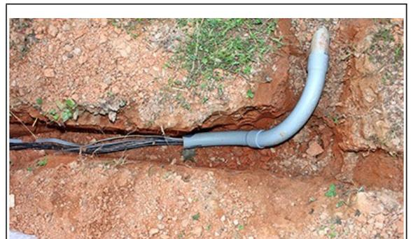
Figure 42: Feed cable conduit into house
