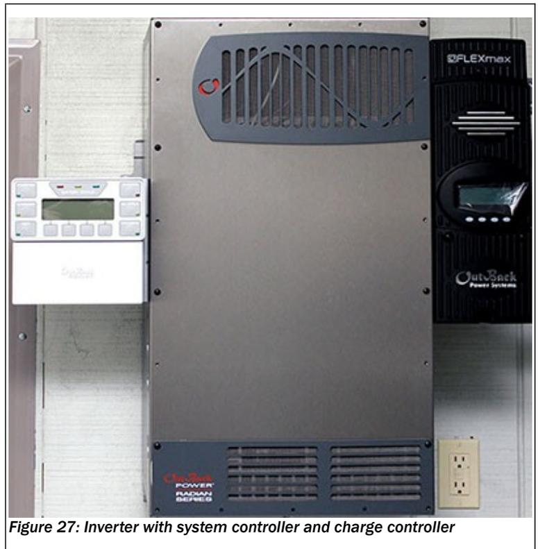
Figure 27: Inverter with system controller and charge controller
