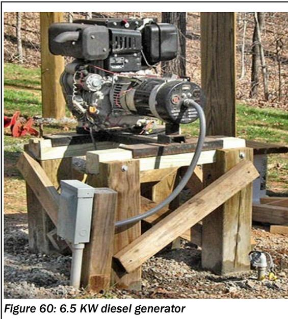
Figure 60: 6.5 KW diesel generator
